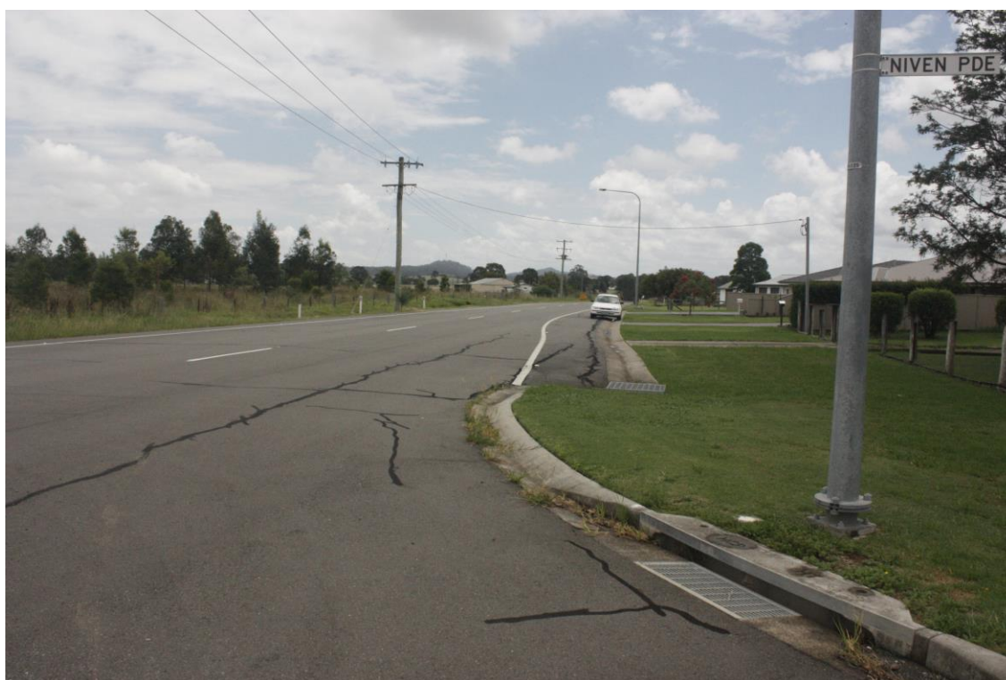
Photo No. 2: Looking right (generally north) along Anambah Road from Niven Parade showing the existing traffic environment and available sight distance.
