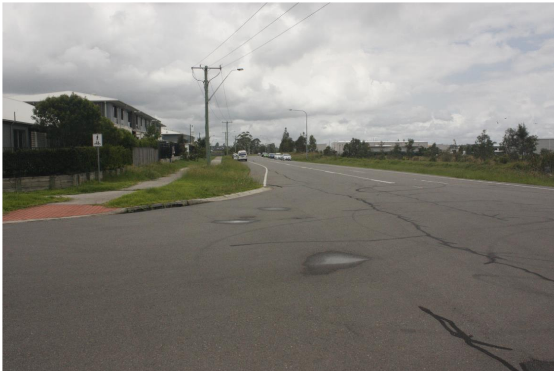
Photo No. 1: Looking left (generally south) along Anambah Road from Niven Parade showing the existing traffic environment and available sight distance.
